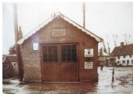
The old fire station
